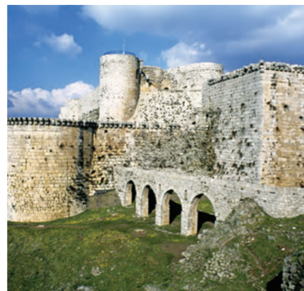
Source 3.68 Krak des Chevaliers in today's Syria, once occupied by Crusader knights, is a concentric castle; note the much higher inner wall.
