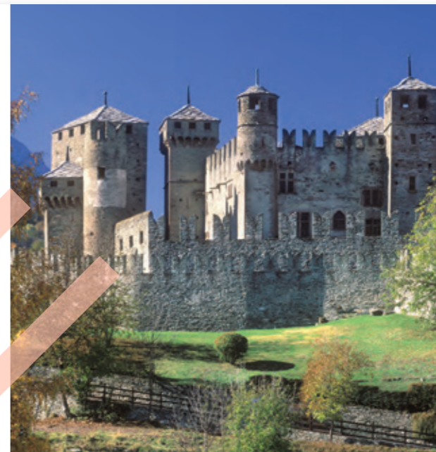
Source 3.67 Fenis Castle in Italy; note the protective outer wall (with its battlements) and the multi-storey keep inside the walls
